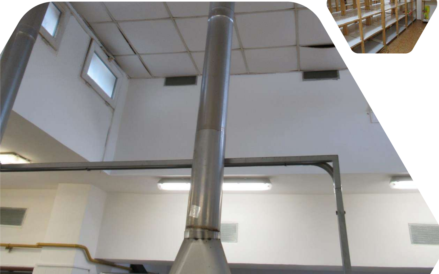
A PREVIOUS KITCHEN
